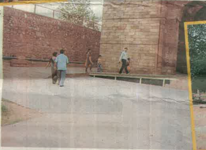
A necessary addition: Ramp in a city monument
